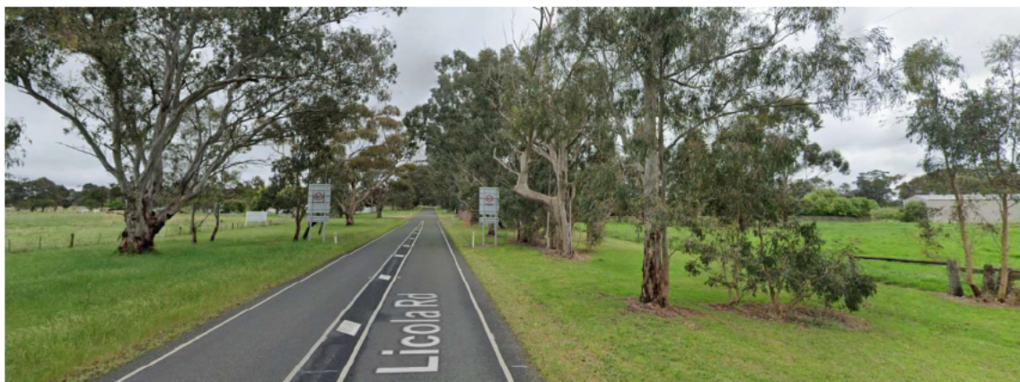
Photograph 1: Looking north along Licola Road. Subject site is on the right of the photograph.
